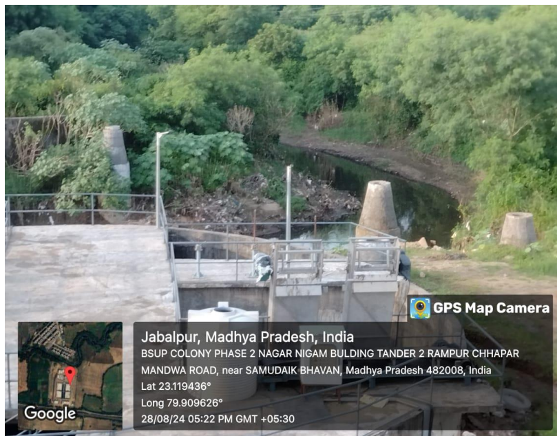
Storm Water Drain
