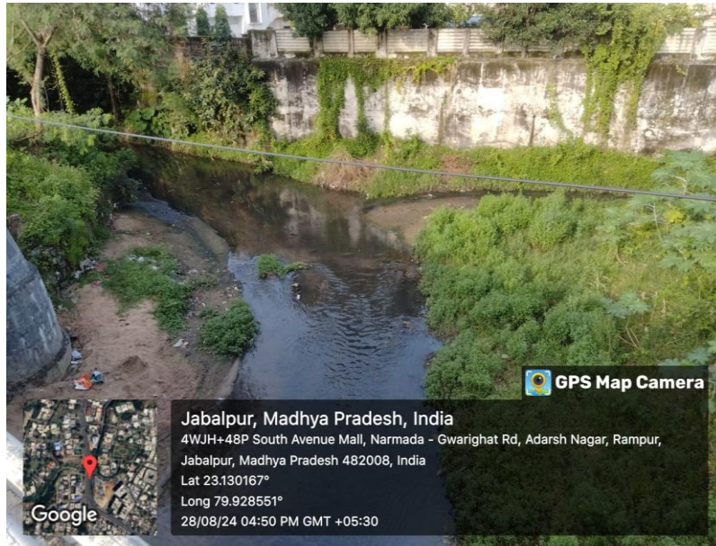
Storm Water Drain
